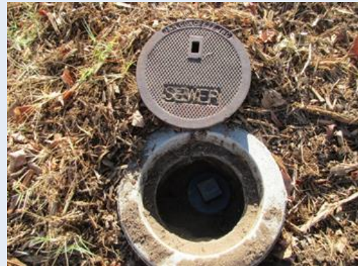
Cleanout access in the front yard
