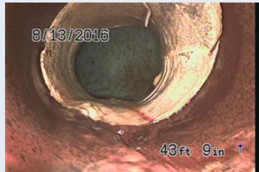
End of the city liner repair
