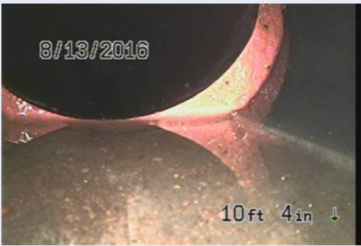
ABS to Clay connection
